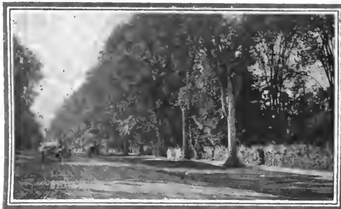
Showing an ideal wide macadam driveway in the Berkshires
